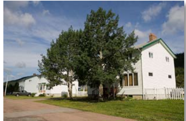
Physicians housing units, Baie Verte
